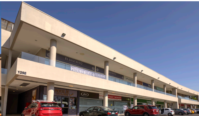
STRIP CENTER SAN CARLOS
